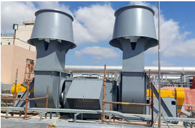
Shown mid-installation, the Model BAIFE 402LV induced-flow high-plume fume exhaust fans at the Sultan Qaboos construction site.
