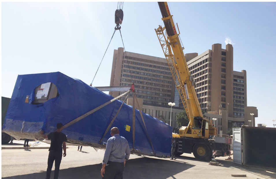
Workers unload one of the new York YVAA Smart Chillers as they are prepared for installation at the King Abdullah University Hospital in Amman, Jordan
