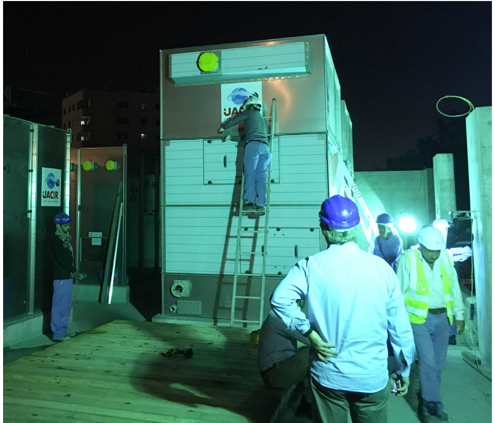
The Energy International crew with help from Jacir-Gohl were able to install the DEWA Data Hub cooling towers in five working days. Shifts were long and tiring extending into the dark of night.
