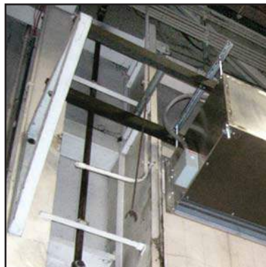
Steel tubing attached to the top of the air curtain can extend to structural supports.
