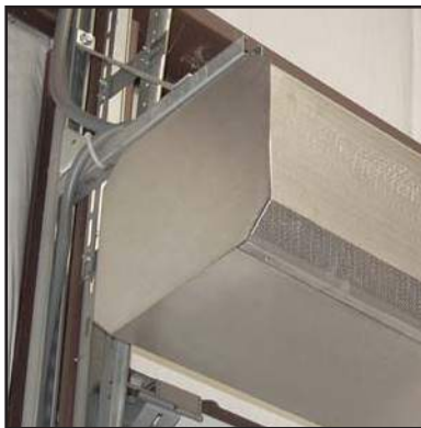
Custom brackets attach to top mounting holes and to wall outside of door track system.
