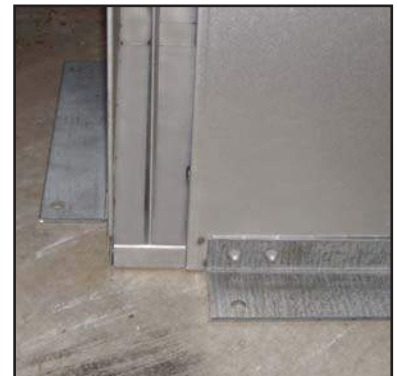
The air curtain can be connected to the floor with brackets and if necessary attached to the wall at top for stability.
