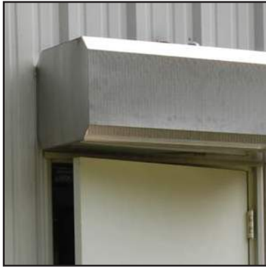
This example shows an air curtain mounted flush with the wall for an exterior application.
