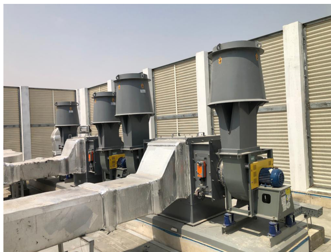
Aisha Bint Hamad SAI Attiya Hospital (above) was built specifically to provide medical care for World Cup fans. Energy International Qatar engineers designed, supplied and oversaw the installation of Twin City Fan high plume fans (left) High plume fans are designed to remove harmful bacteria- and germ-laden from the hospital building.
